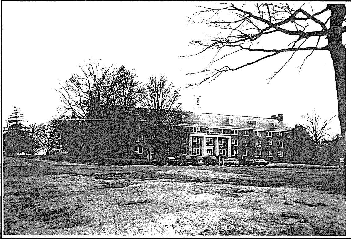
Photo ID: Building 307, East Facade, 4/97
