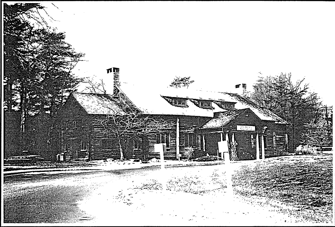
Photo ID: Building 302, East and South Facades, 12/97
