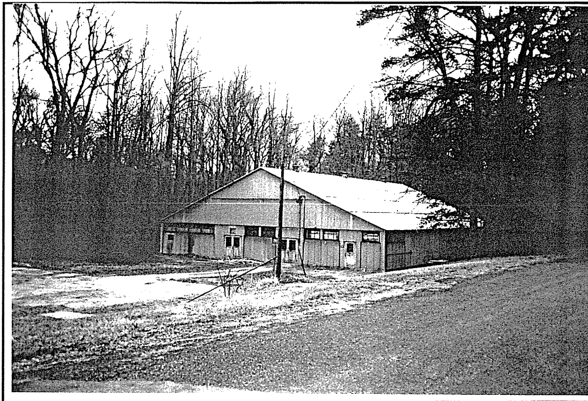
Photo ID: Building 421, South and East Facades, 2/26/97
