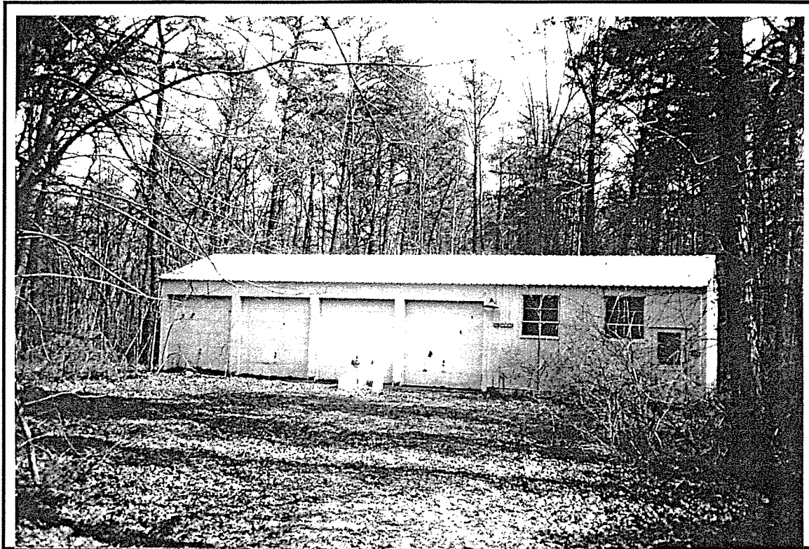
Photo ID: Building 472, West Facade, 2/26/97
