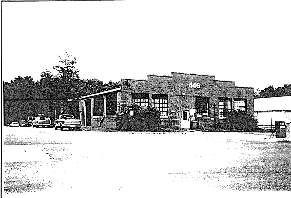
Photo ID: Building 446, South and East Facades, 2/20/97
