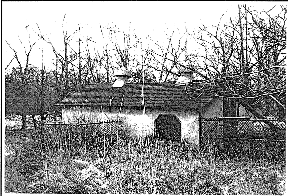
Photo ID: Building 341R, West and North Elevations, 5/97
