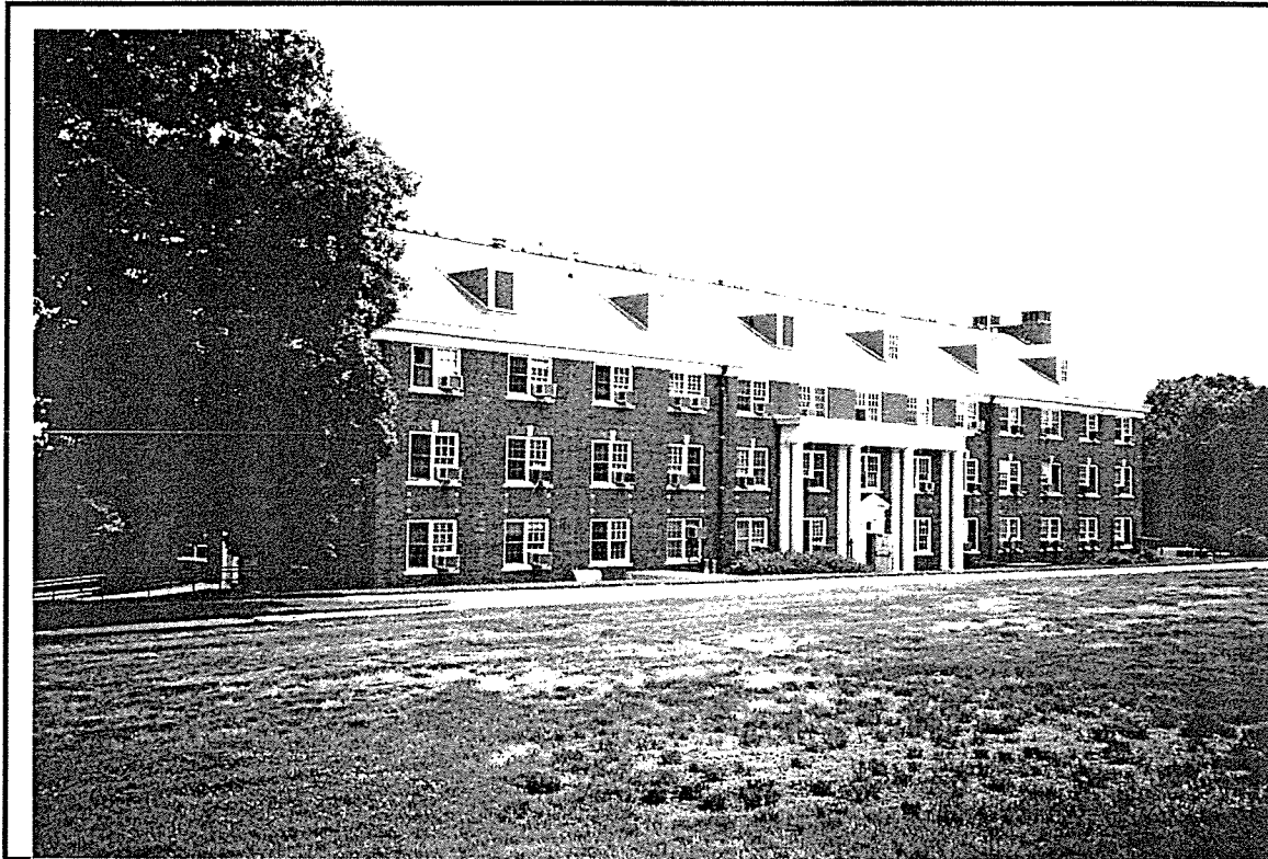
Photo ID: Building 306, West Facade, 6/97
