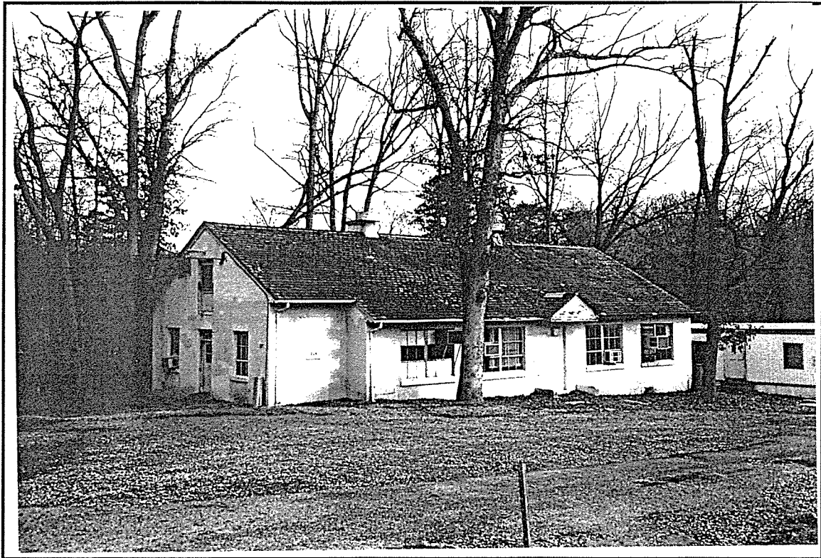
Photo ID: Building 334, South and West Facades, 4/97
