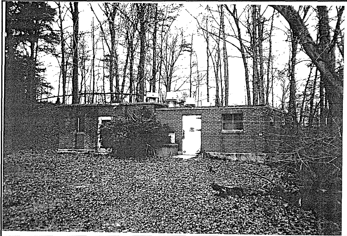
Photo ID: Building 315, South Facade, 4/97
