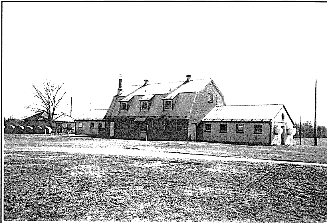
Photo ID: Building 434, North Facade, 2/21/97
