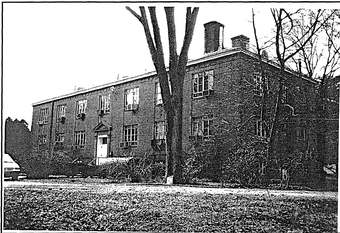
Photo ID: Building 476, East and North Facades, 2/26/97
