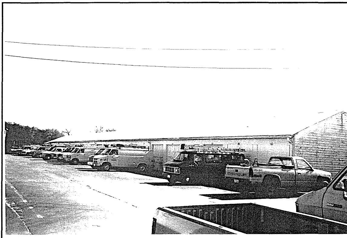
Photo ID: Building 427, North Facade, 2/20/97
