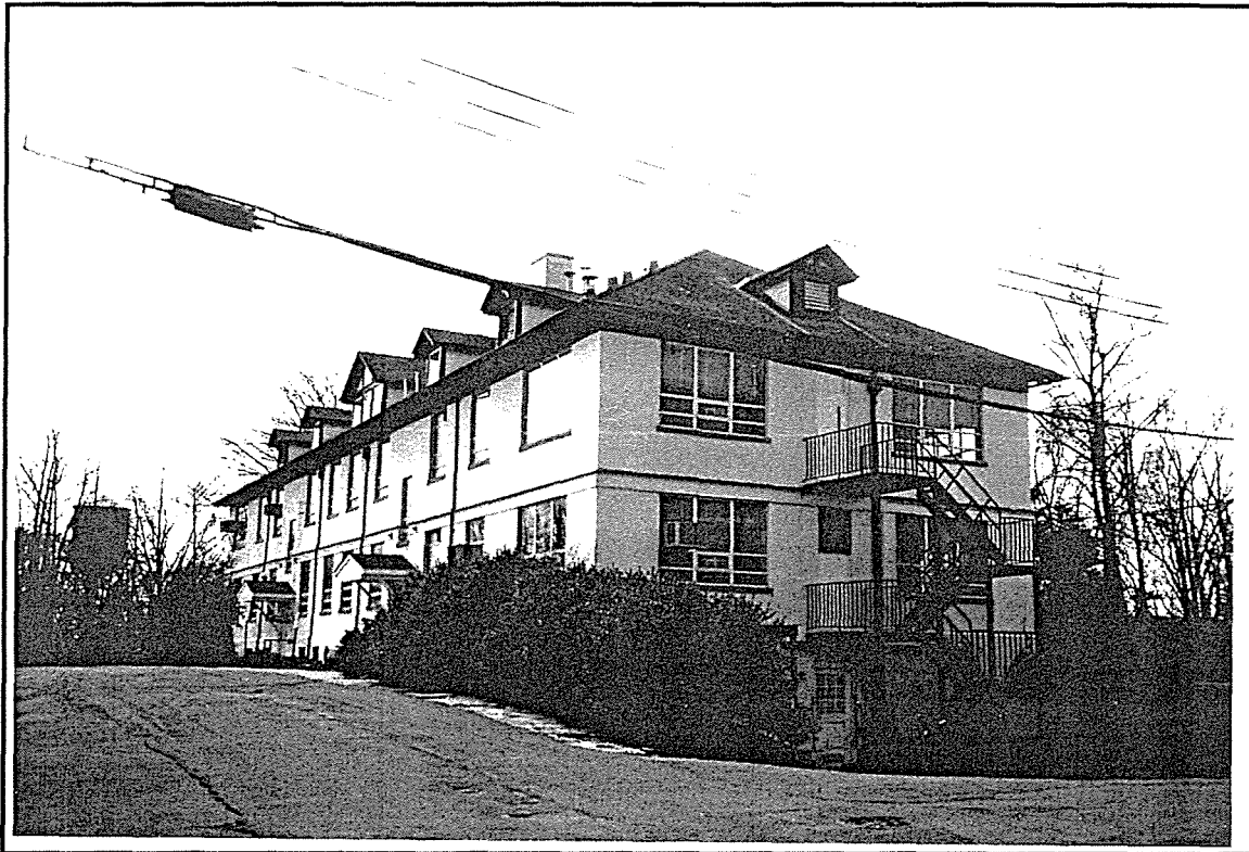
Photo ID: Building 318, North and East Facades, 4/97
