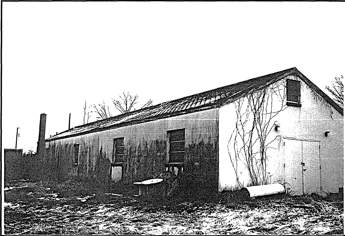
Photo ID: Building 327, North and West Facades, 12/97
