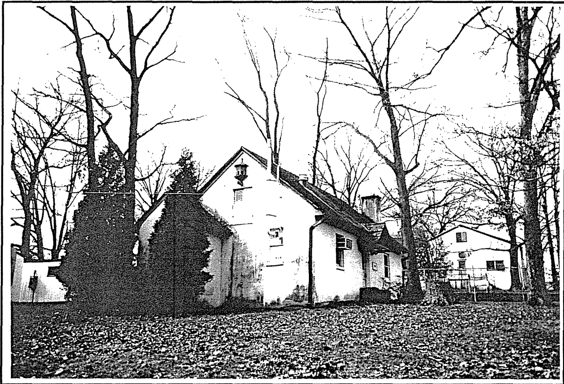
Photo ID: Building 328, North and East Facades, 4/97
