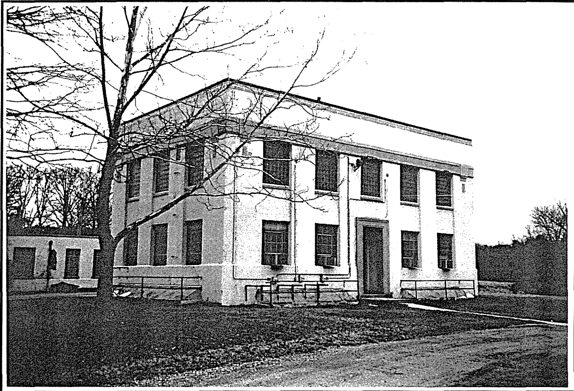
Photo ID: Building 402, South and West Facades, 2/26/97
