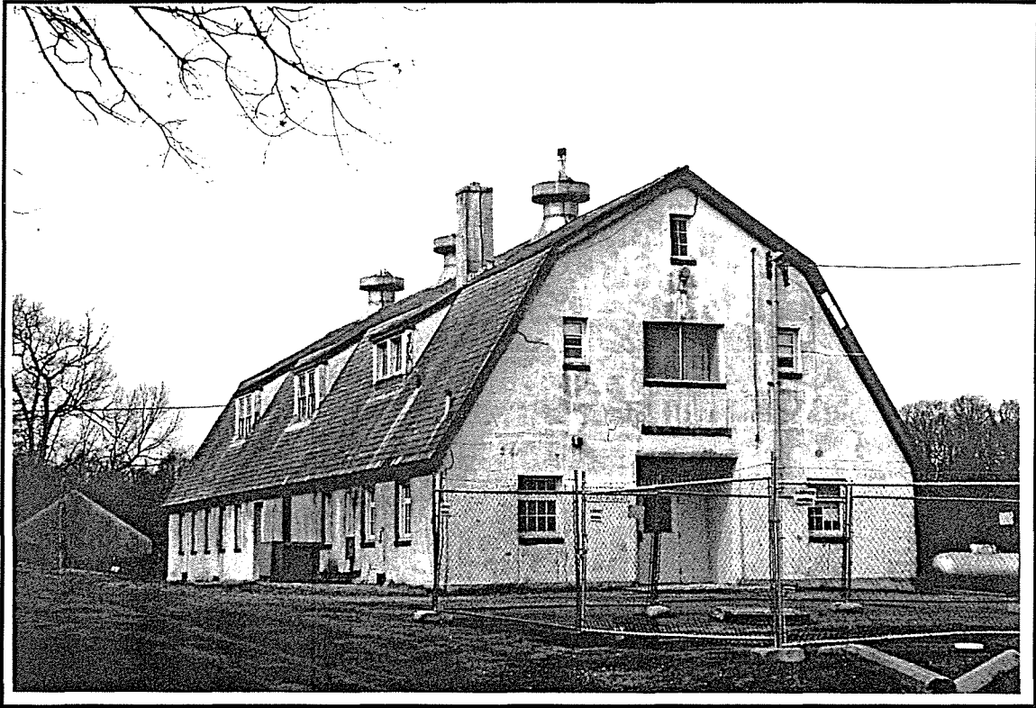
Photo ID: Building 322, East and South Facades, 4/97
