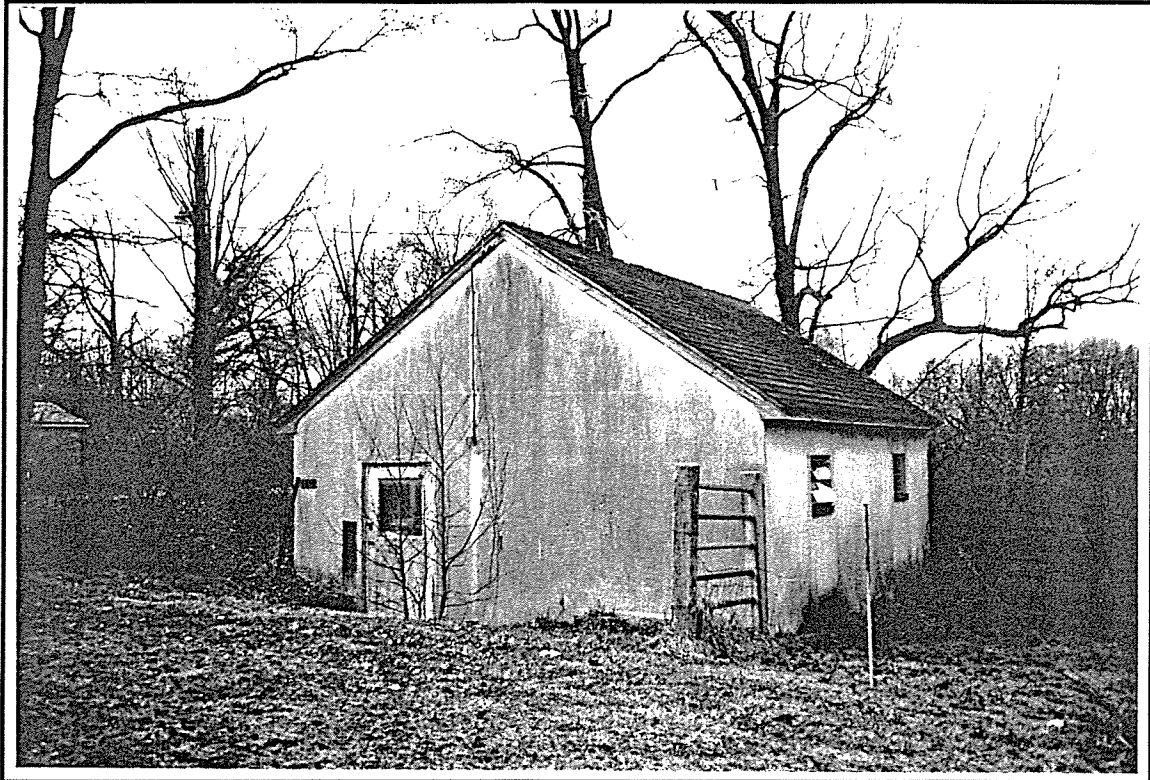
Photo ID: Building 323, North and East Facades, 4/97
