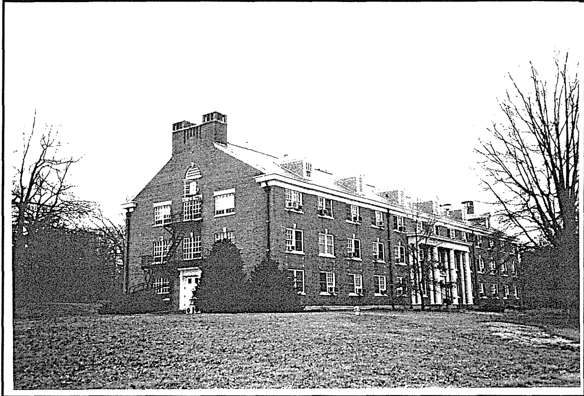
Photo ID: Building 308, East and South Facades, 4/97
