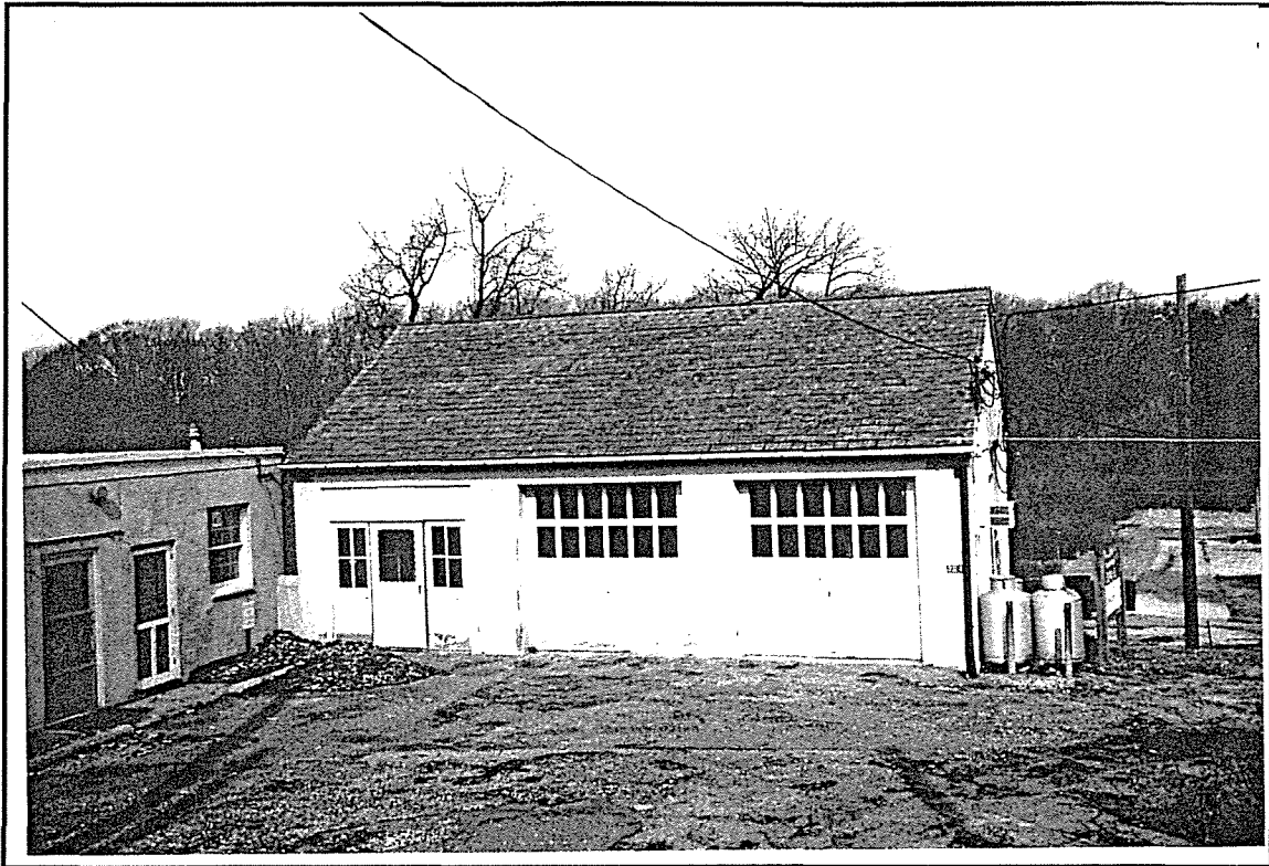
Photo ID: Building 324, South Facade, 4/97
