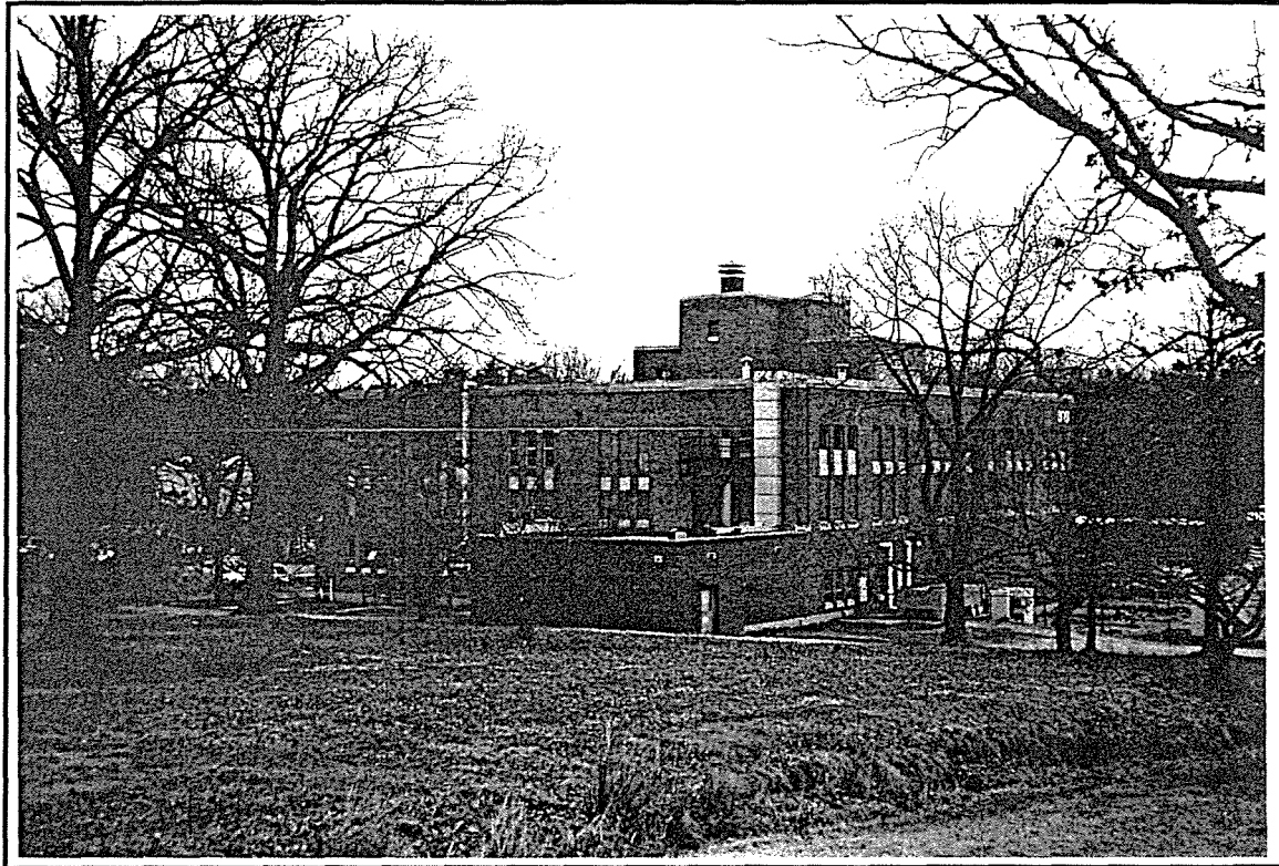
Photo ID: Building 309, South and West Facades, 4/97
