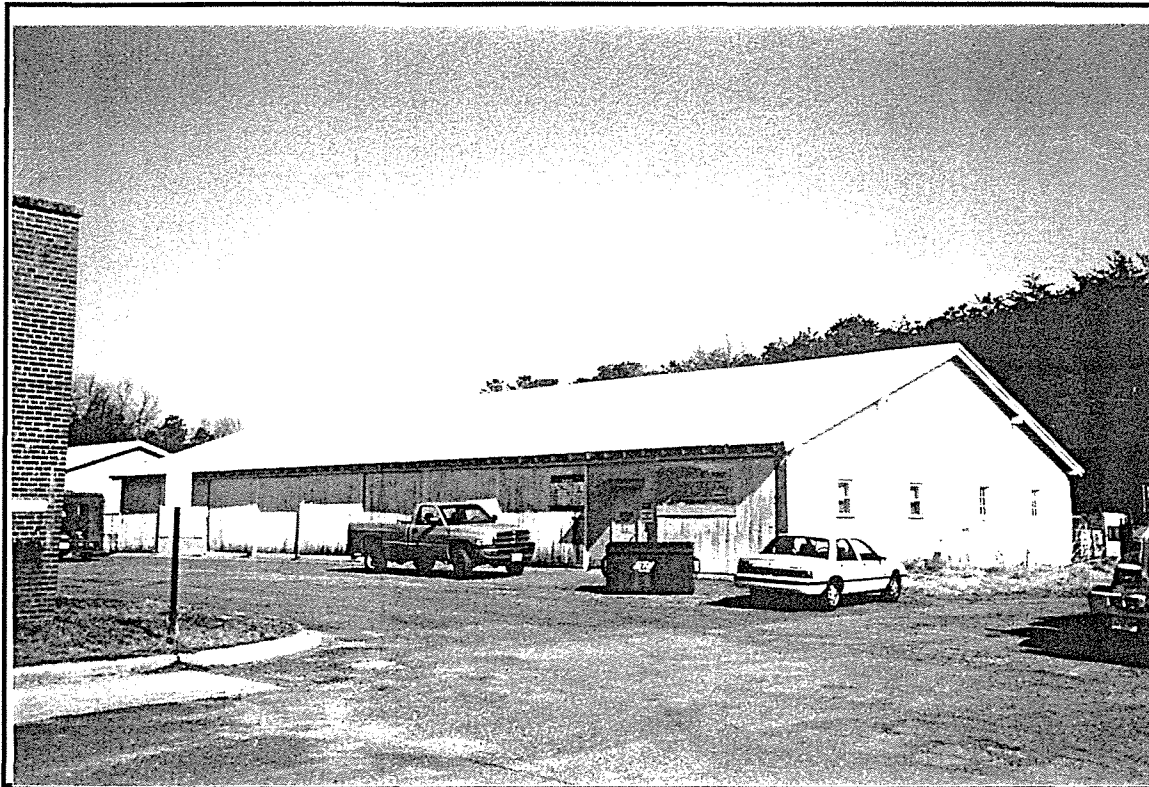
Photo ID: Building 449, West and South Facades, 2/20/97
