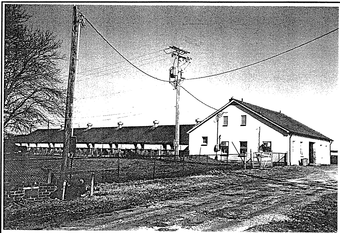
Photo ID: Building 536, West and South Facades, 2/20/97
