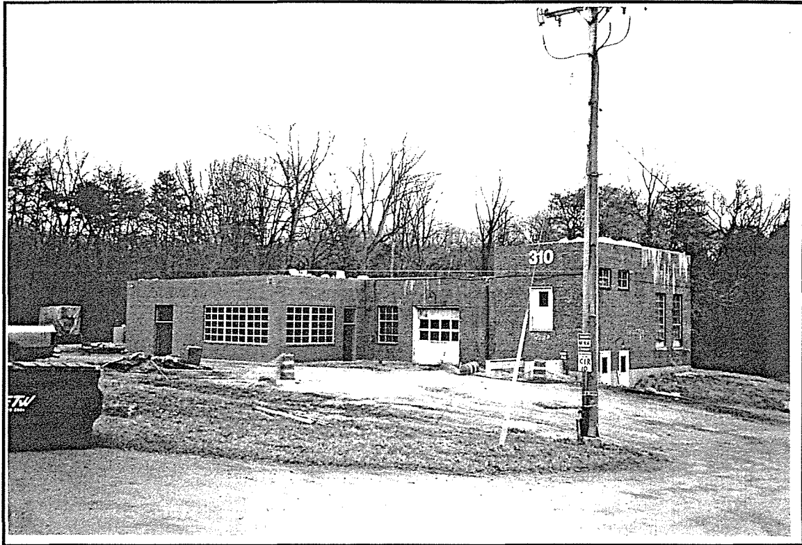
Photo ID: Building 310, South and West Facades, 4/97
