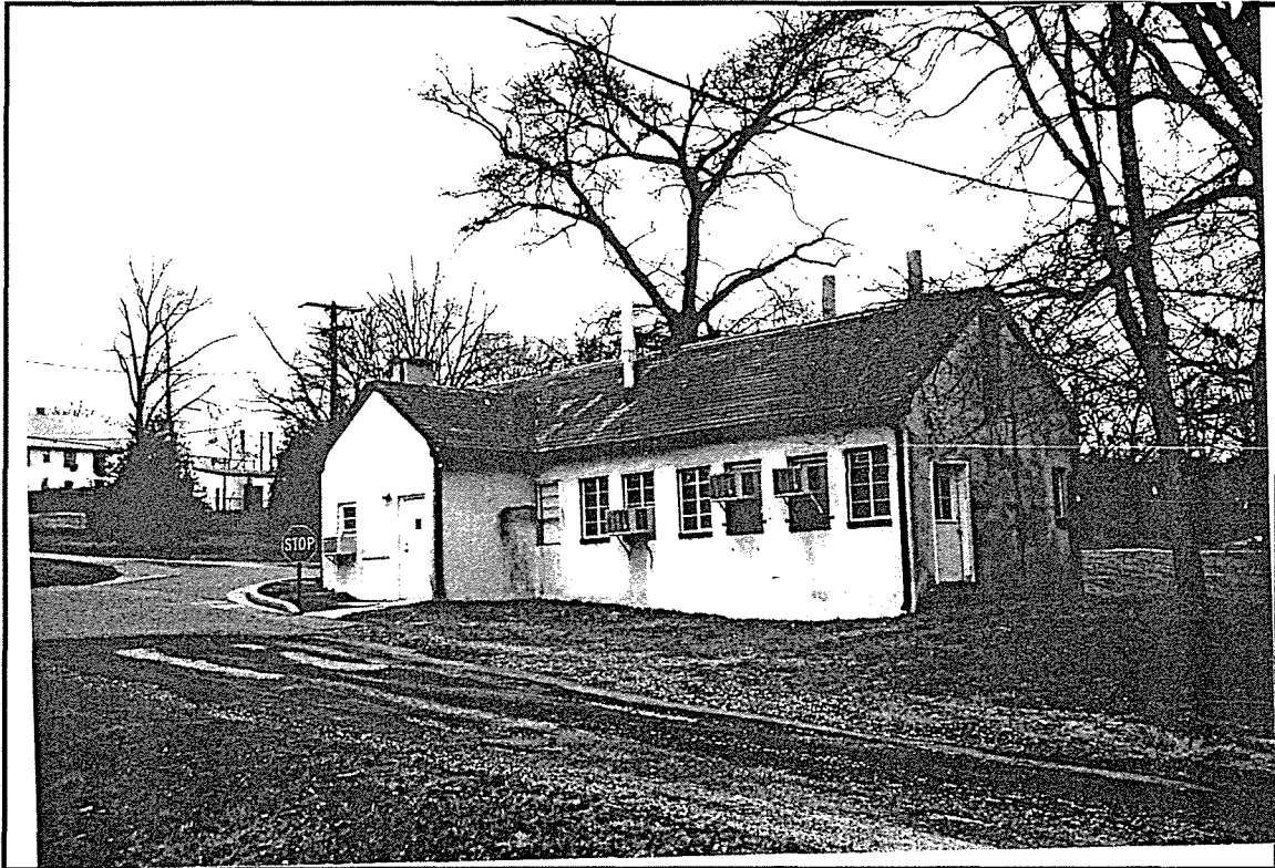
Photo ID: Building 338, East and South Facades, 4/97
