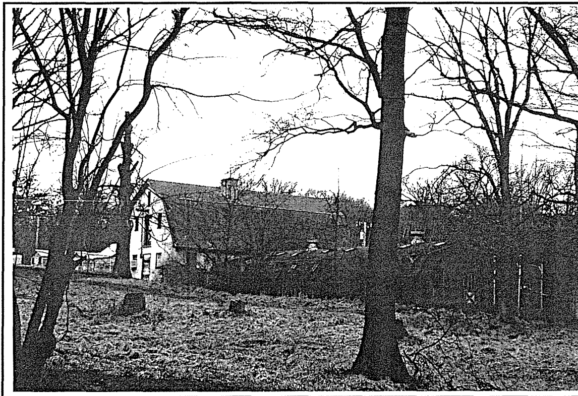
Photo ID: Building 340, East and South Facades, 4/97
