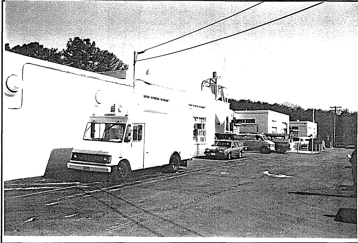
Photo ID: South Facade, Building 426, 2/20/97
