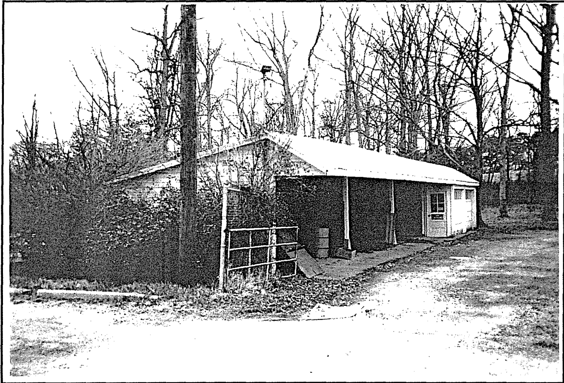
Photo ID: Building 411. South and East Facades, 2/26/97
