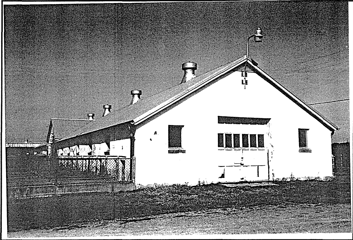
Photo ID: Building 537, South and West Facades, 2/20/97
