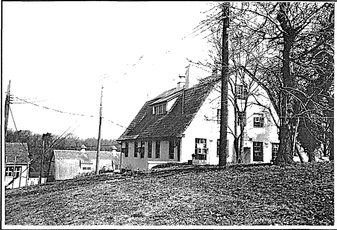
Photo ID: Building 321, South and West Facades, 4/97
