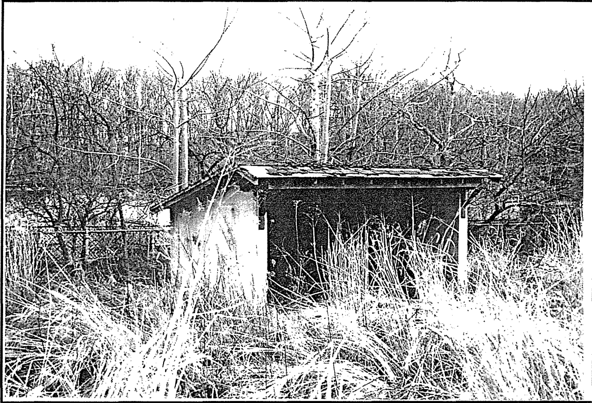
Photo ID: Building 342A, South and West Facades, 12/97
