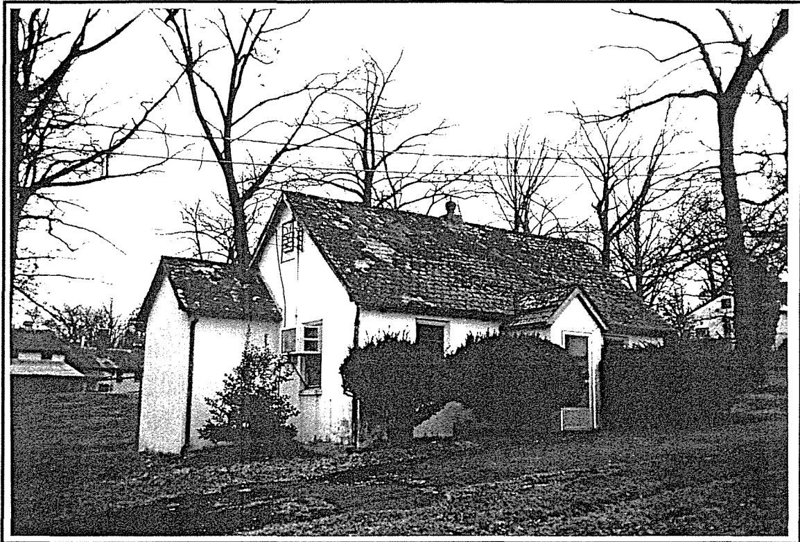
Photo ID: Building 357, North and East Facades, 4/97
