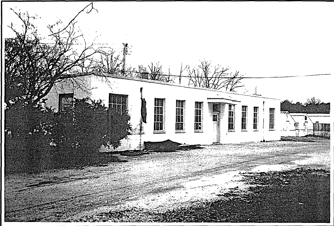
Photo ID: Building 404, South and West Facades, 2/26/97
