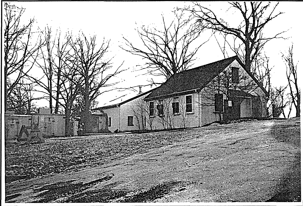
Photo ID: Building 321, West and North Facades, 4/97
