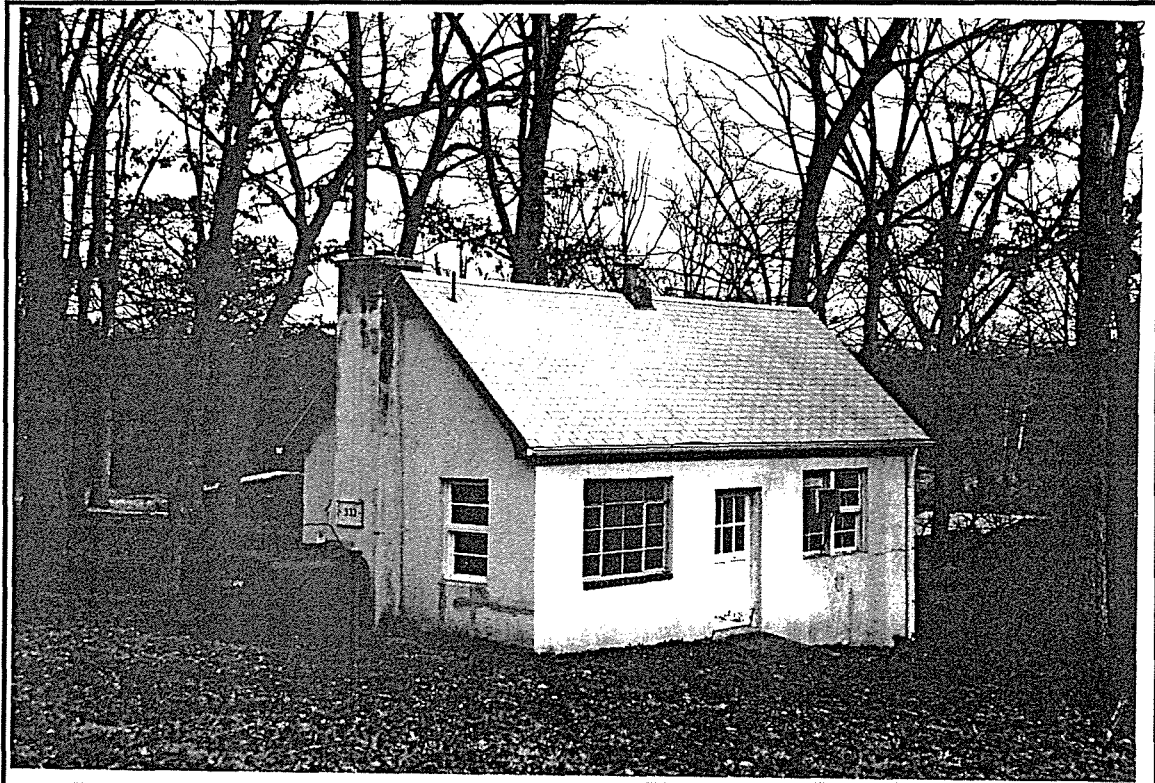
Photo ID: Building 333, South and West Facades, 4/97
